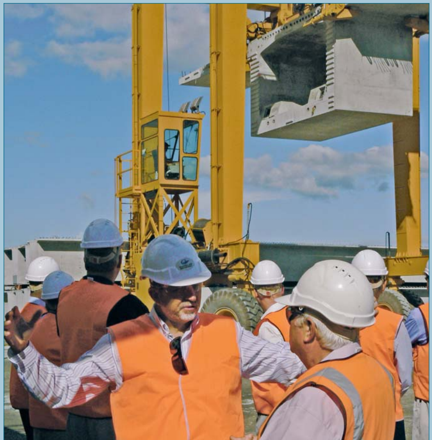
Queensland Motorways hosted a visit by members of the ARF Board in February to inspect progress on the massive Gateway upgrade project in Brisbane. Board members are pictured at the Eagle Farm precast yard producing the concrete elements for the second Gateway Bridge, currently under construction by the Leighton Abigroup Joint Venture.
